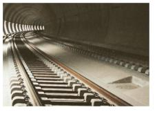
Rubber boots and pads have been initially developed for biblock sleepers with connection bar and have been used in several Swiss tunnel constructions such as Bötzberg, Grauholz, Mattestetten-Rothrist and in different railway stations: Zürich, Kloten and Lausanne. Rex elements were inserted in the project of different metro lines abroad: Brazil, Egypt, Greece, France and Italy.
