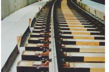
Having different possible applications in the field of the railtracks for undergrounds and tramways, Rex Articoli Tecnici SA produces boots and the microcellular pads with a static and dynamic stiffness that are remarkably interesting. Vibration damping may either occur through the application of special rubber pads or by employing special profiles, optimised by means of simulation, which the company can execute in its own laboratories.
