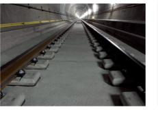
Biblock sleepers without connection bars of the LVT type have been used in the projects pertaining to the new transversal line crossing the Alps (Zimmerberg, Lötschberg and Gotthard). This system is widely used abroad (The Channel Tunnel, Hong Kong, Taiwan, Brazil and the USA).
